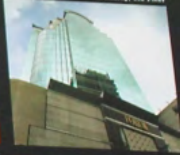
Mexico City—FORUM Building, 4th Floor
