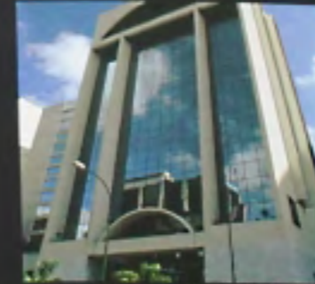
Caracas—Torre Nord Building, 2nd Floor
